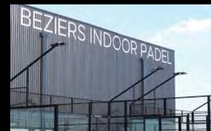
Padel court BIP (Béziers Indoor Padel)
